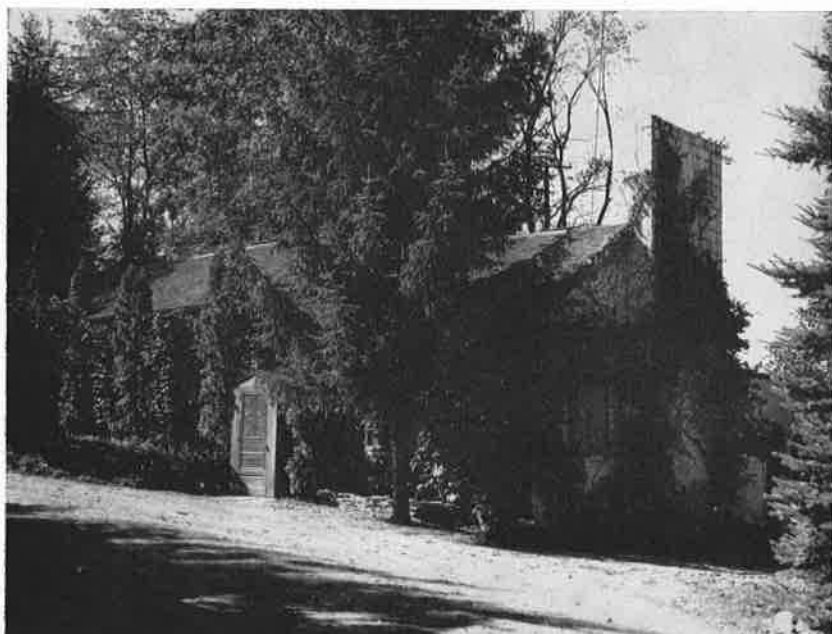
Maintenance Supervisor's House
