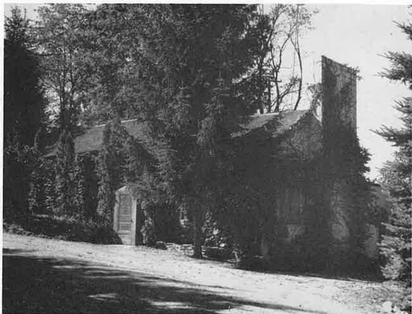
Maintenance Supervisor's House
