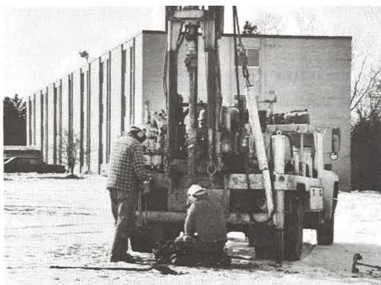
Workers conduct soil-borings on the site of the new residence halls.
