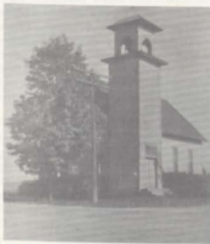
BUILDING BEFORE REMODELING
