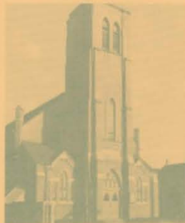
The Old Building
