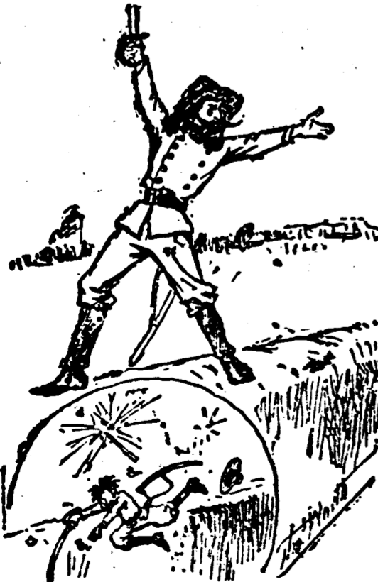
BEFORE AND AFTER THE SHELL EXPLOSION.
